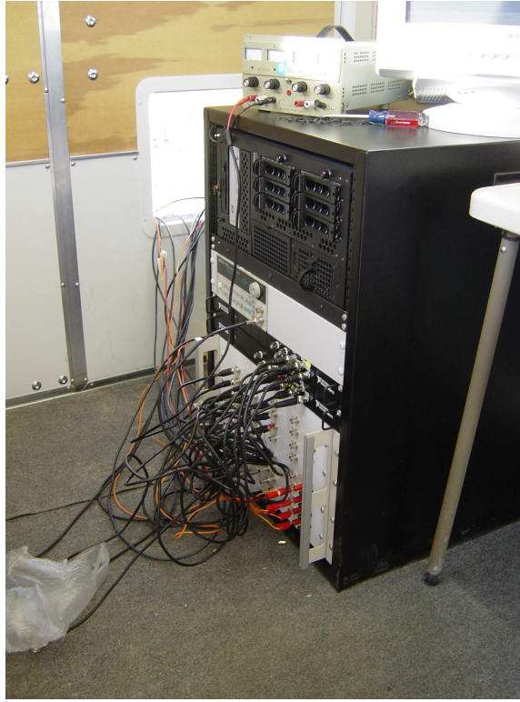
Figure 3.5: Shows all the power and signal cables attached to the receiver box during a field experiment.
